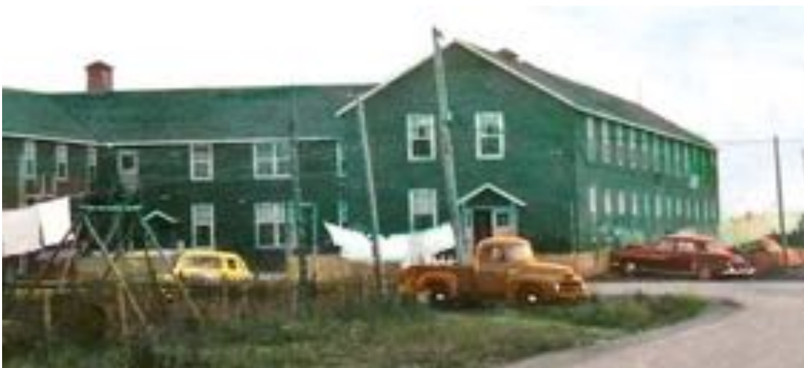
Typical cars near bldg 108 Fosse Avenue
