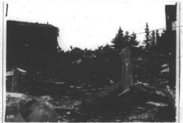
Construction Shack Fire
